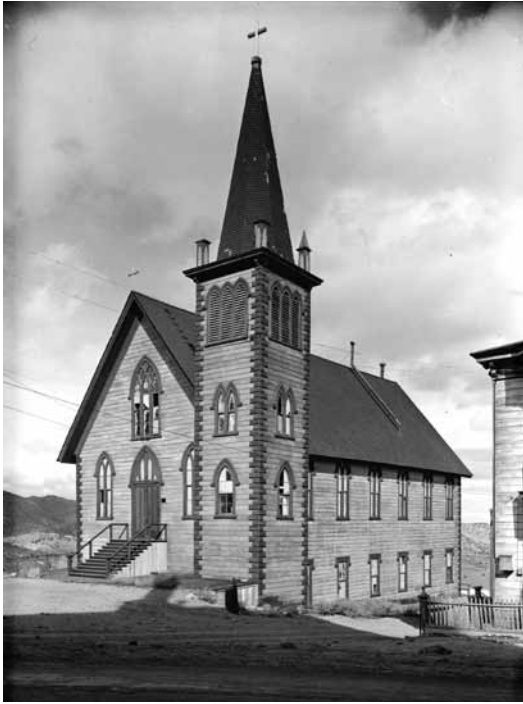
FIGURE 12 (left). St. Paul's in 1936. Note the replaced doors and stair rail. Photograph by Robert Kerrigan of the Historic American Buildings Survey. ( Library of Congress )
